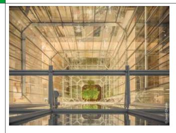
Glass developed a technically complex insulating glass construction for the corners. The 28 double cylindrically curved rectangular panes ranged in dimension from 1638 x 5546 mm to 1663 x 3440 mm. The 44- and 46-degree bends each form a 90-degree corner with a flat section in between, followed by a short straight section after the bends.
