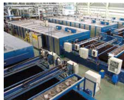
Cold End Coating System & Cooling Fan Racks
