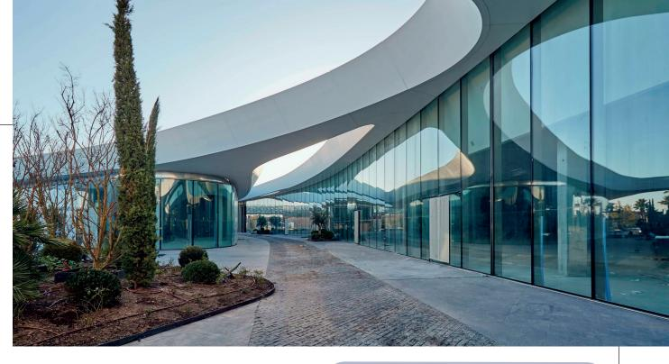
tempered and laminated glass, were used to ensure maximum safety. The Tvitec 6 metres of curved glass for Martifer brings together great elegance with the ecoefficiency of double-glazing.
