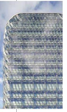
light to enter the building as well as full indoor climate control, especially in winter. Tvitec supplied around a thousand metres of glass for the project, half of which was tripleglazed. tempered and laminated with a unique solar control coating from Glastroesch, namely Combi Neutral 61/32 with Low Iron. Laminates were also produced for large balustrade areas.
