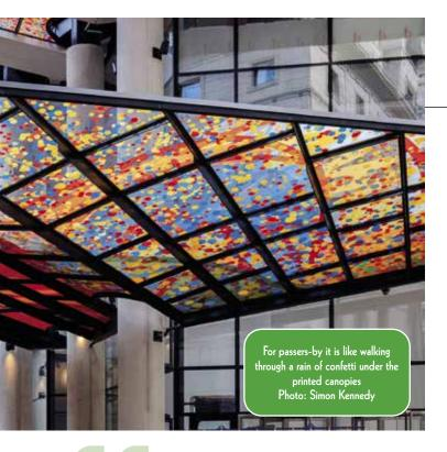
double layer safety glass made from 8 mm low-iron (heat-strengthened glass) with digital printing. Artwork in position 2 or 3. As the art extends to the façade, there are also printed insulated glass panes. These are each made from two double laminates (6 mm heat-strengthened glass). They are filled with argon and printed in position 2 or 7. In total, sedak supplied 149 laminates and 370 insulated glass panes.
