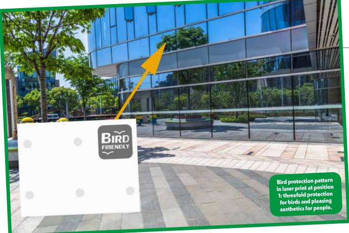
cess and the system enable the imprint to be applied without having to remove or replace the glass panes. The mobile printing device is attached to the facade so that the pattern can then be revealed. "Sustainability and bird protection are now more relevant than ever before," Rainer asserts. "There is great interest in such a solution, especially for public, commercial and prestigious buildings, as
