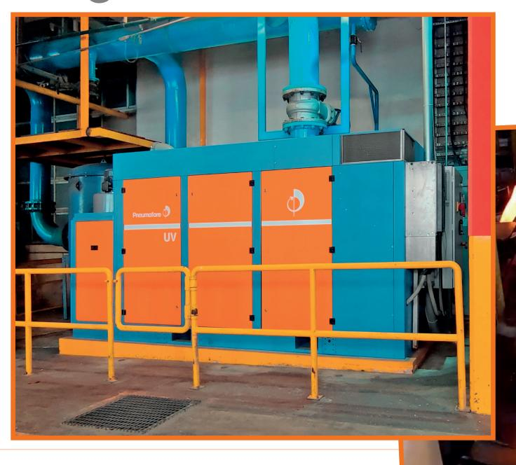
A leader in the manufacturing, distribution and sale of beer in Mexico and part of A.B. InBev, the world's largest beer brewer, Grupo Modelo recently installed its third PNEUMOFORE UV100 Rotary Vane vacuum pump at the company's Tierra Blanca plant.
