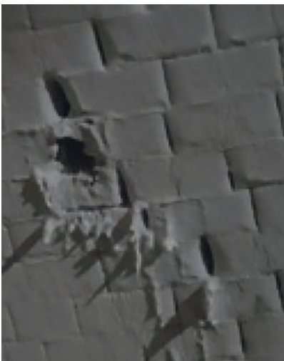
Standard degradation with silica crown © SEFPRO, All rights reserved 2026
