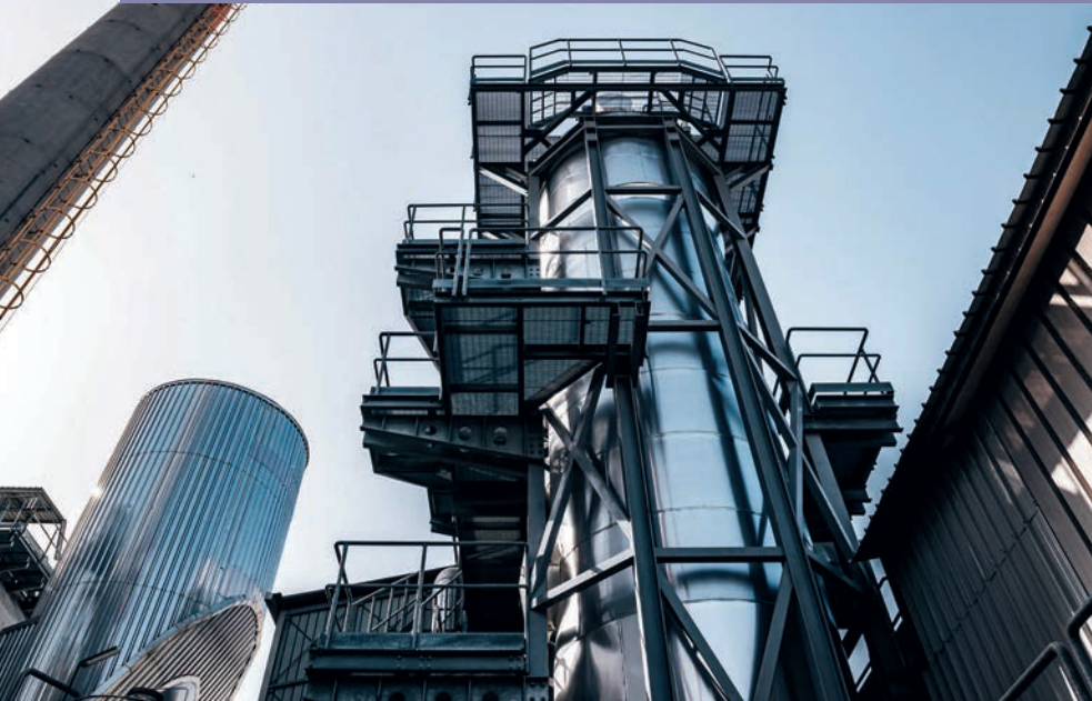
Pic. 3 - example of Stara Glass double-shell recuperators for Centauro furnaces
