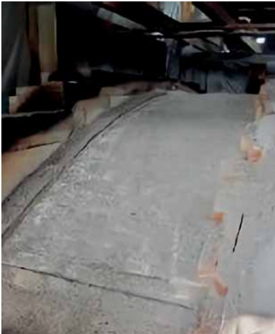
Fig 10. Complete sealing and insulation of the melting crown with Compac Sol and insulating mixes
