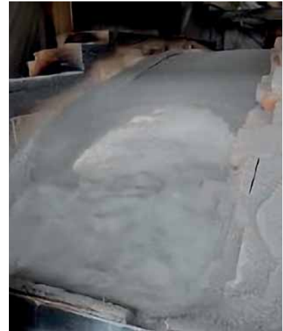
Fig 10. Complete sealing and insulation of the melting crown with Compac Sol and insulating mixes
