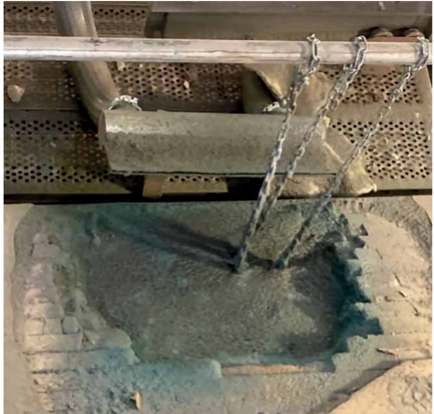
Fig 9. Sealing of the repaired area with hanging bricks with Compac Sol
