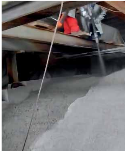
Fig 10. Complete sealing and insulation of the melting crown with Compac Sol and insulating mixes
