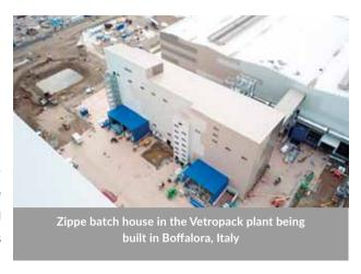
The order was processed by Zippe on a turn-key basis. The project comprises all parts, including steel construction, erection, pipework, cabling, commissioning as well as training of Vetropack personnel. The batch house is designed to supply two melting furnaces.
