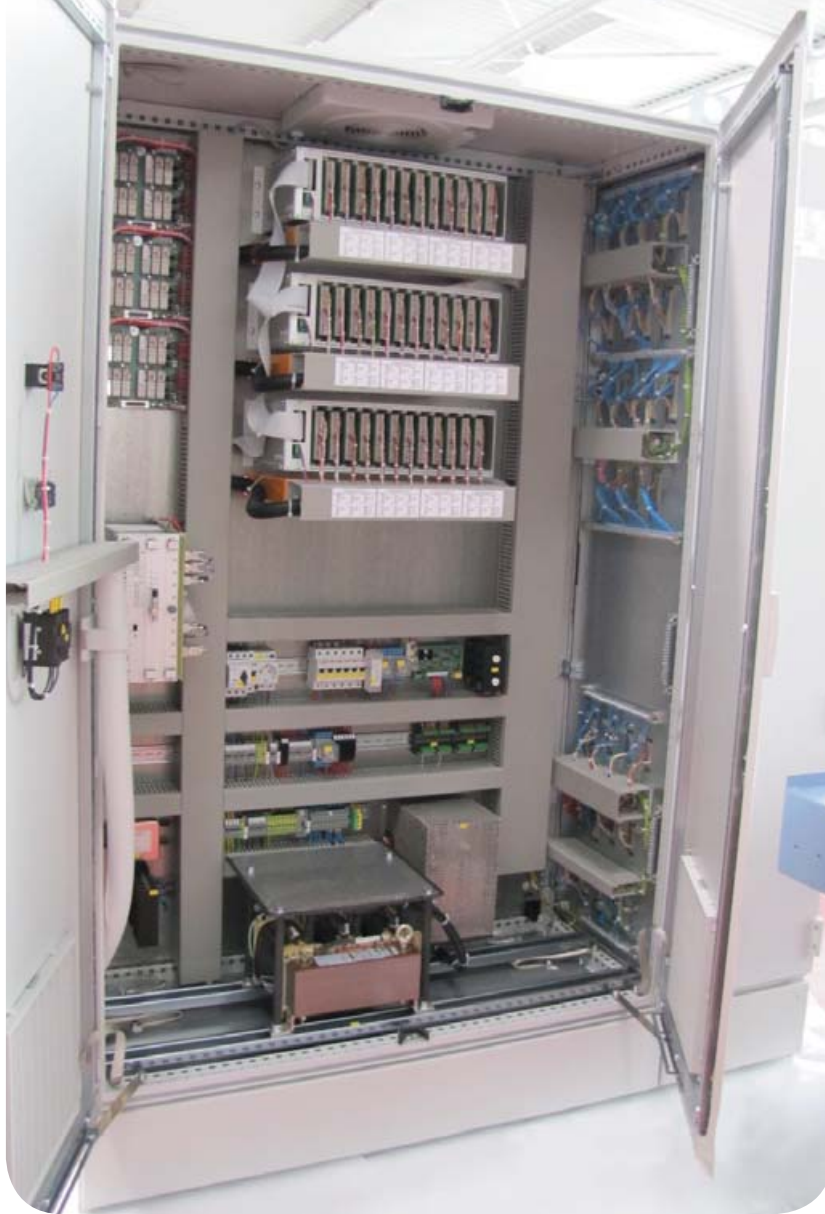
Neat and tidy: this (new) control cabinet still houses an original EPRO control (left). Each retrofit should also include new cables, depending on the system's age and condition. They could become brittle over the years and lead to faults in view of the harsh production conditions prevailing in glassworks
