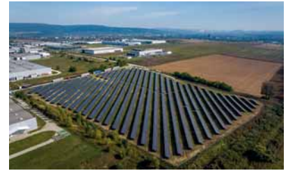
The solar farm operated by E.ON provides AGC Glass Hungary with a source of renewable energy
