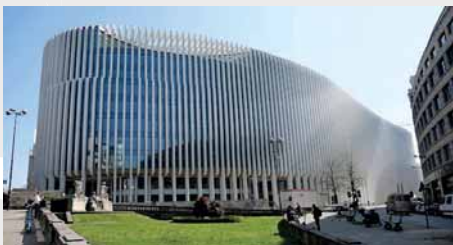
In the façade, "Stopray Ultra-60 on Clearvision" ensures high daylight transmission, effective sun protection, thermal insulation and colour neutrality - Photo: AGC Glass Europe
