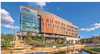
Solarban® 70 glass, red brick, limestone masonry and metal display a high-tech facade at the University of Texas at San Antonio (UTSA) National Security Collaboration Center - Photography: Tom Kessler
