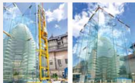
For the glass pavilion, six panes from Finnglass measuring 2.4 by 12.5 metres and weighing 2.8 tonnes had to be set vertically into grooves.
