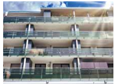
Glass balustrades with integrated green-transparent OPVs that generate energy on the building in Stuttgart Möhringen - Copyright: ©ARMOR ASCA
