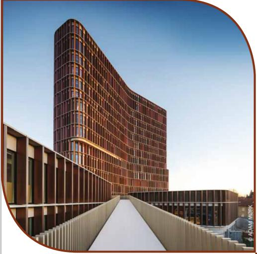
breaker. The shutters that have in some cases been designed as movable elements act in accordance with the weather. Where there is a large amount of sunlight, copper grids automatically protrude from the slats. They reduce the energy input, but still allow daylight to enter the rooms. The material of copper was not chosen by chance, but by way of an homage to the surrounding architecture with the traditional brick facades.
