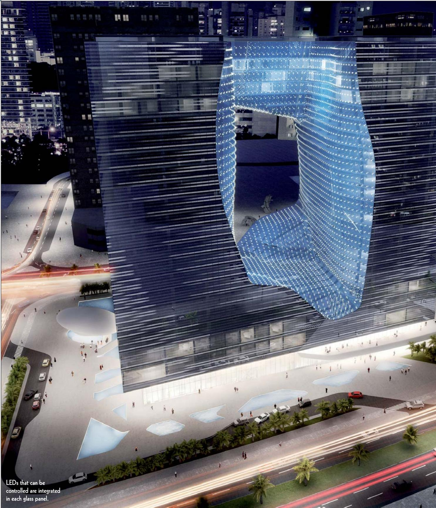
LEDs that can be controlled are integrated in each glass panel.
