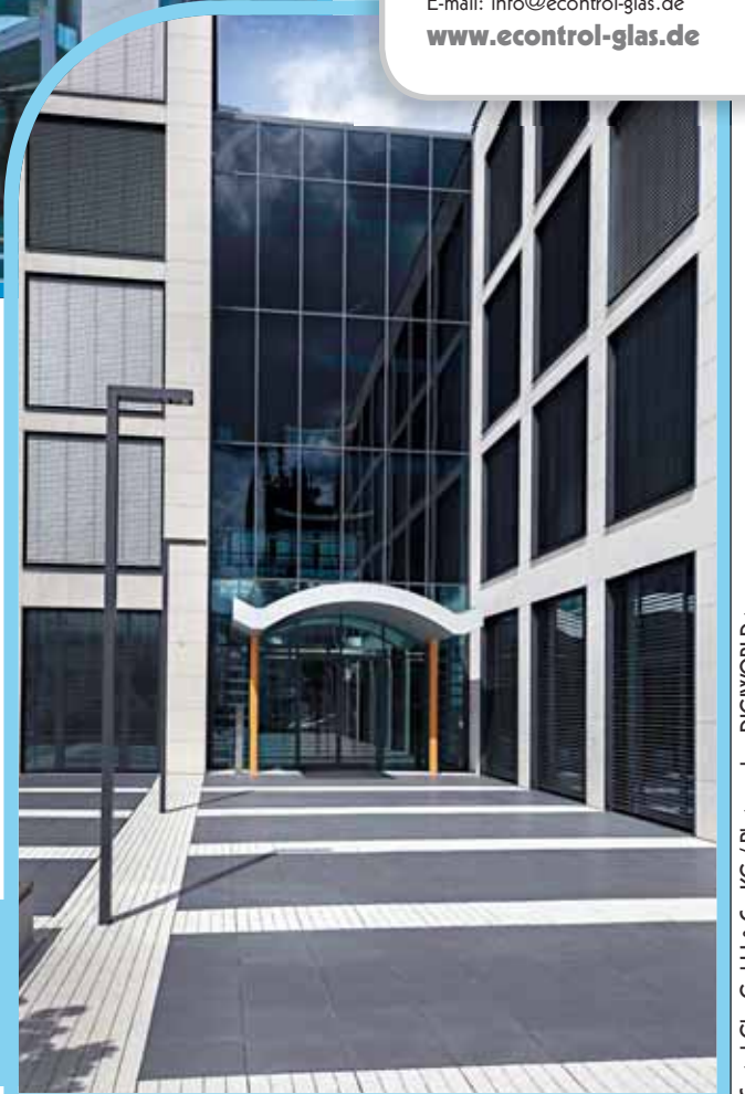
The 16-metre-high glass atrium connects the two wings of the European headquarters. Even at the highest dimming level enough daylight enters the interior of the building
